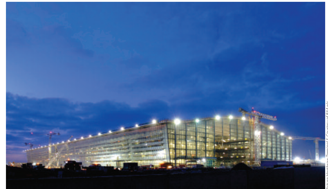
Picture: Heathrow Terminal 5. Courtesy of BAA plc
