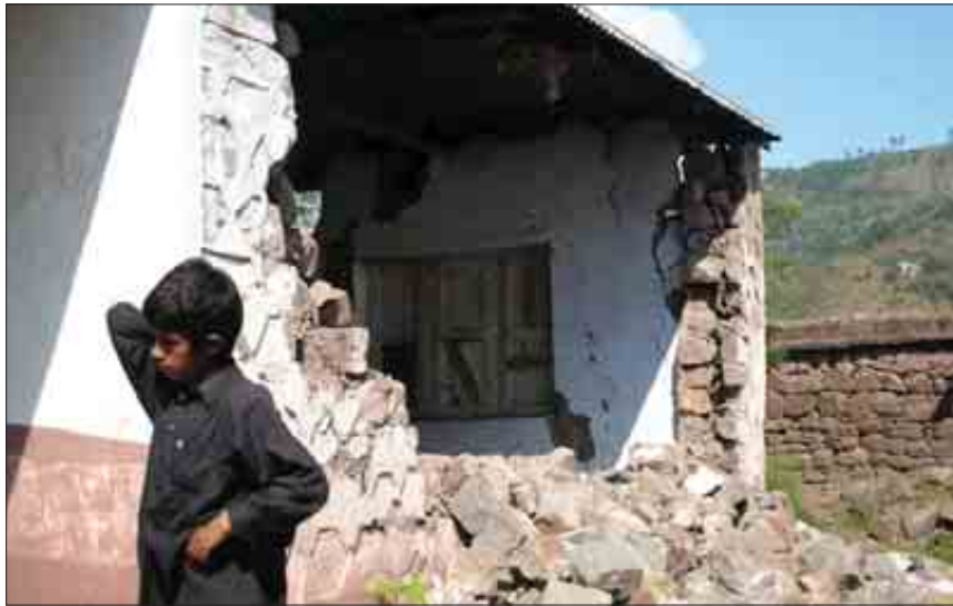
Earthquake Reconstruction, Pakistan, Kashmir Schools Rebuilding project © Arup
