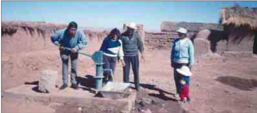
Final stage of commissioning a new well, drilled by YUNTA in a school playground in Papel Pampa, Provincia Villarroel
