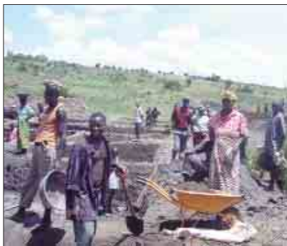
Dam Construction - using readily available equipment and providing local employment
