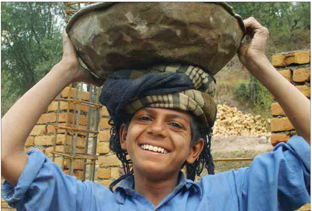
Earthquake Reconstruction, Pakistan, Kashmir Schools Rebuilding Project © Arup
