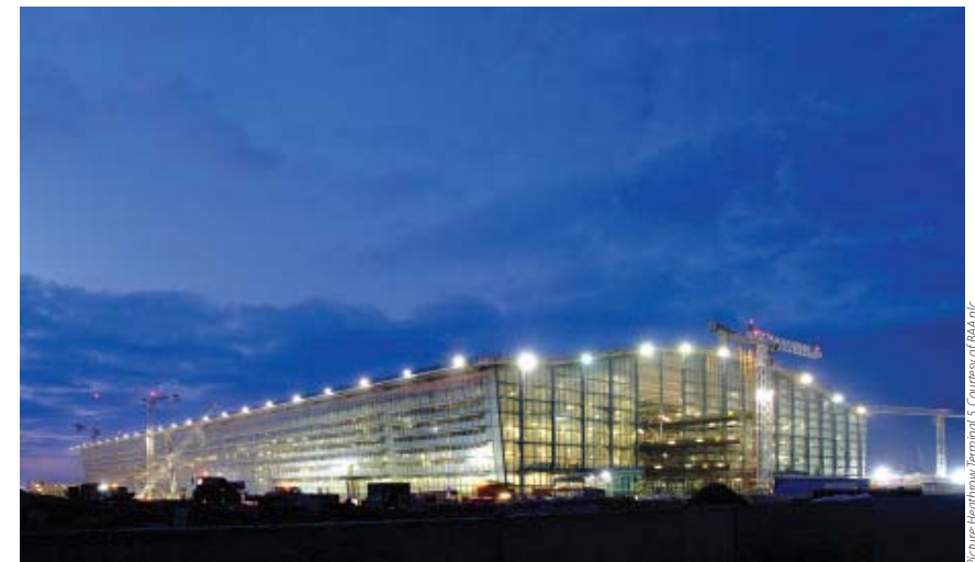
Picture: Heathrow Terminal 5. Courtesy of BAA plc
