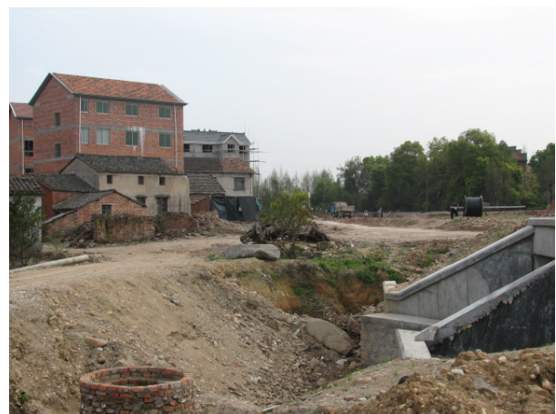
Figure 2 undercrossing make up for the breaking former road
