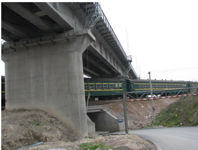
Figure 3 potential safety hazard in sharp turn
