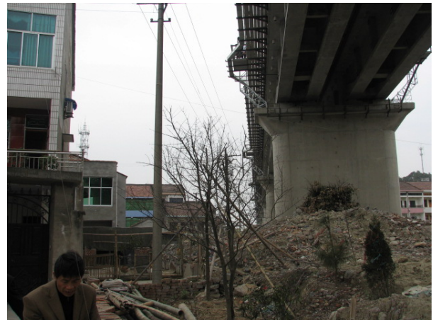
Figure 1 viaduct through the villages
