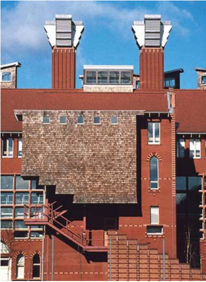
The Queens Building for the School of Engineering and Manufacture at De Montfort University, by Short Ford Architects with Max Fordham LLP as environmental engineer, is a masterpiece of legible design. Designed to be naturally ventilated and daylit the results are explicit in the architecture. The engineering workshops are lit with roof lanterns whilst the tall chimneys induce sufficient draught to naturally ventilate the lecture theatres.
