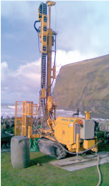
Figure 10: drilling borehole for ground-source heat pump
