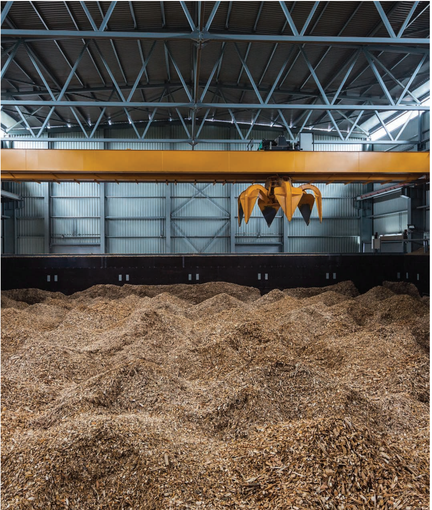
Storage of wood chips
